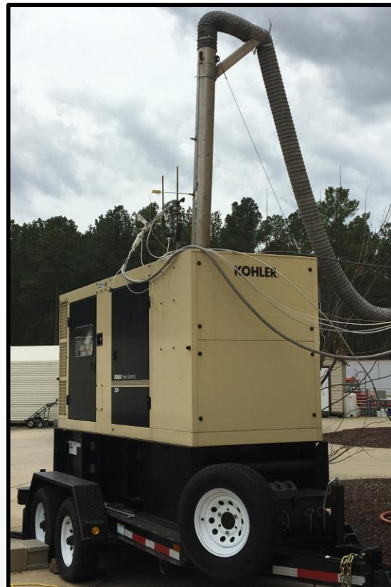
Stationary Diesel Facility (200kW genset)
